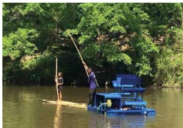
Figure 3 Water turbine transport (Chula-Pidthong 4), showing the incorporation of indigenous knowledge using a bamboo raft to transport the turbine
