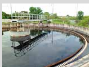
Non-oxygen biological wastewater treatment system (activated sludge)
